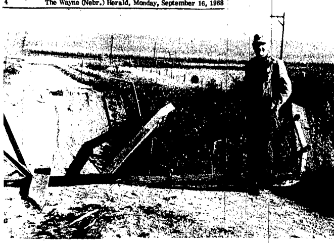
THE STRAW THAT BROKE . . . Joe Erikson of Wakefield, superintendent of the fourth district in Dixon County, seems a bit puzzled about the collapse of this bridge on a county road just three-quarters of a mile north of Concord. Erikson said they were not sure when the bridge collapsed or who drove over it. The county was informed of the collapse Thursday. Built about 50 to 60 years ago, the bridge is a suspension bridge and probably was intended for nothing over 15 tons. It will cost under $5000 to replace the bridge, according to county officials.
